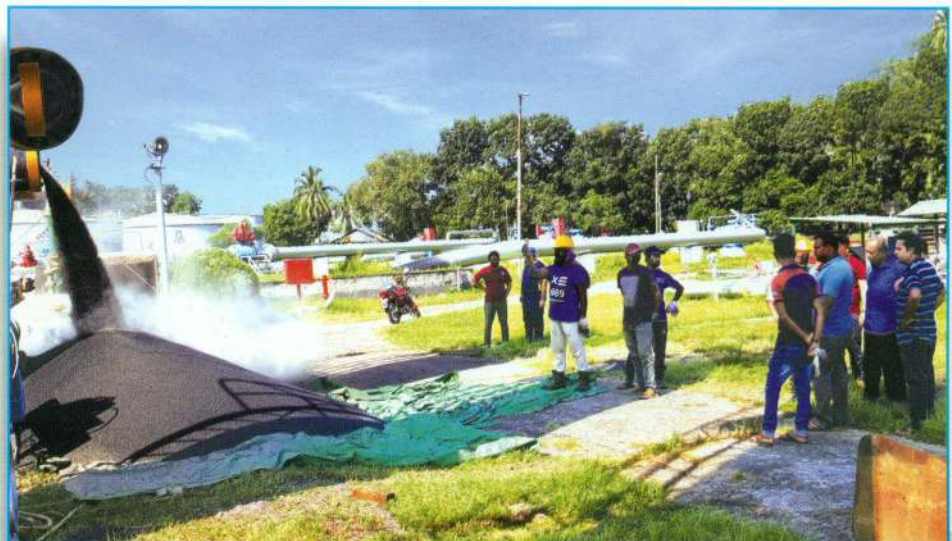
Replacement work of Silicagel of gas process plant at Bakhrabad Field.
